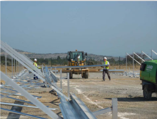
Installation des structures
